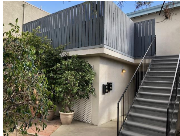
Tenant's Front Doors and Unit Access
