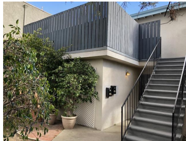
Tenant's Front Doors and Unit Access
